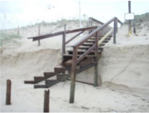
Dorian caused significant beach and dune erosion at the **108A Ocean Blvd** dune crossover and destroyed the ocean side stairs
